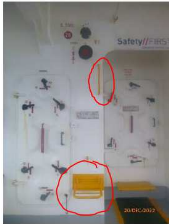
Step and hand hold installed on bulkhead
